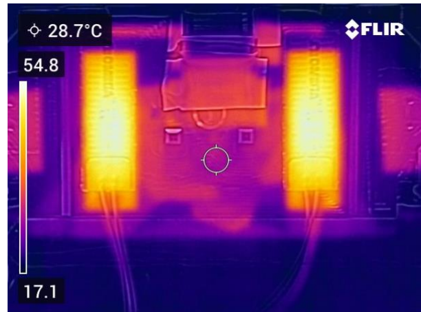
Figure 8: Tank Heater Verification by FLIR
