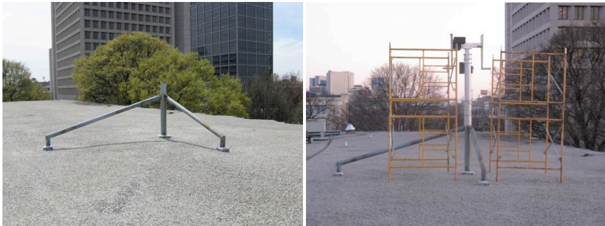
Figure 22: Pictures of the pre-existing structure and the mounting of the rotor system.
